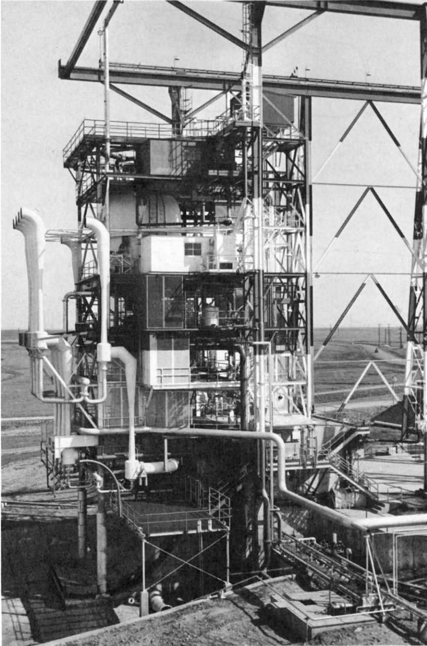
Fig. 3 Saturn S-IVB Stage Six Engine Firing Program in Progress at Sacramento, California
